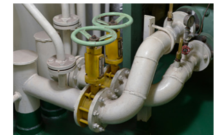
Seawater mains and pipes
